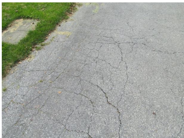
Chapel Court alligator cracks and edge deterioration
