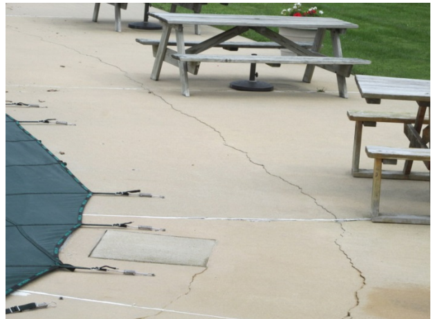
Significant pool deck cracks
