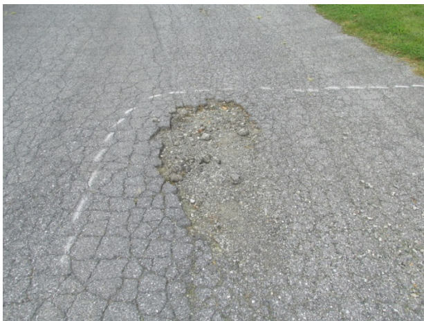
Hedgerow court alligator cracks and pothole
