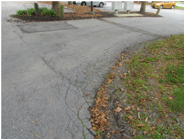
Wyndham Court previous patches, alligator cracks and edge deterioration
