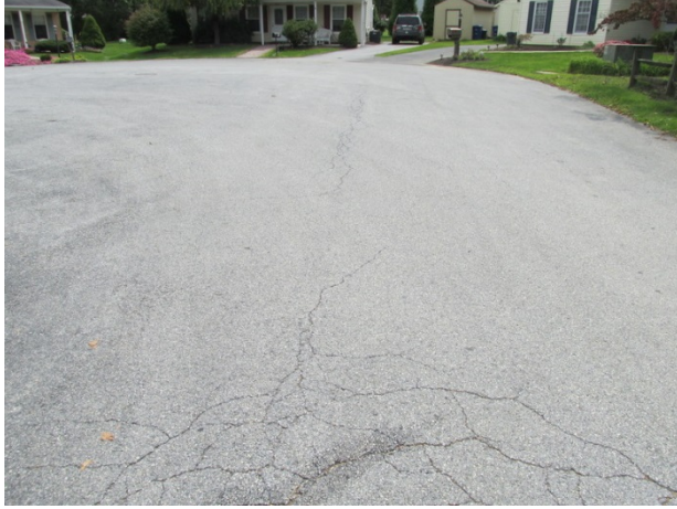
Essex Court alligator cracks and deterioration
