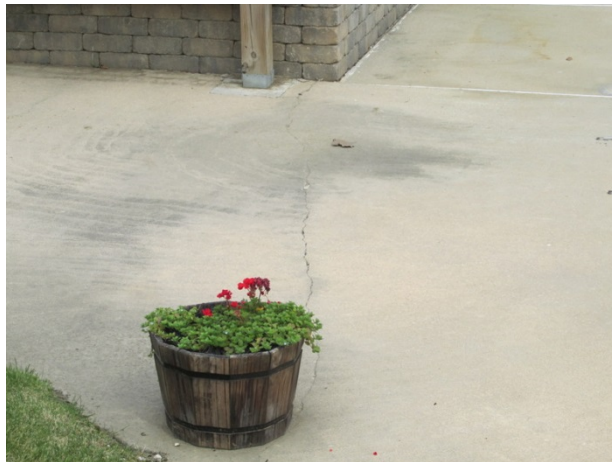
Pool deck crack
