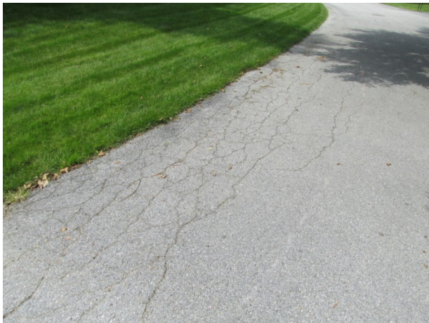
Suffolk Court alligator cracks and edge deterioration
