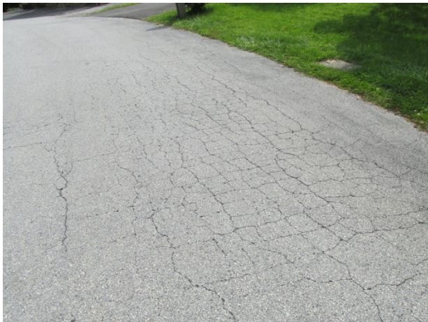
Canterbury Court alligator cracks
