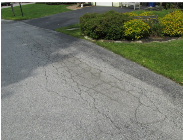
Somerset Court alligator cracks and edge deterioration
