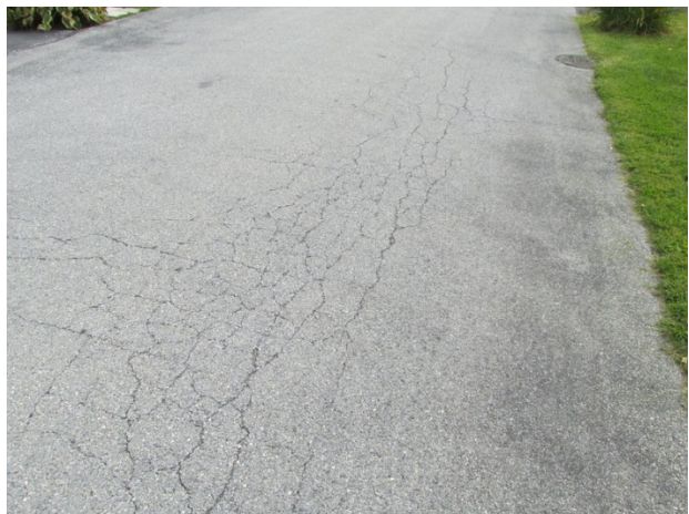
Windmere Court alligator cracks
