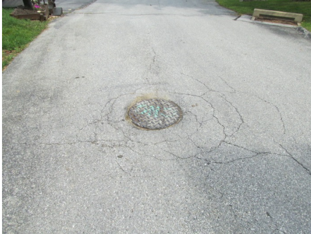
Settlement and alligator cracks at manhole
