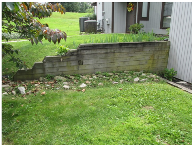
Timber retaining wall
