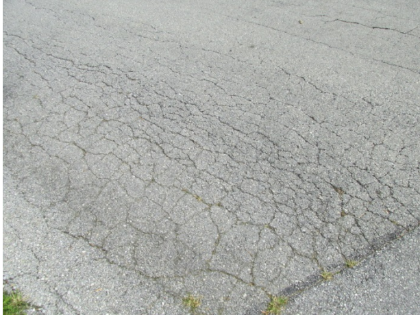
Gloucester court alligator cracks
