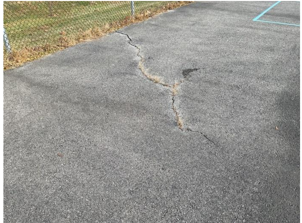
Surface cracks
