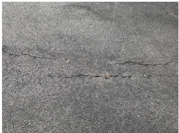
Surface cracks
