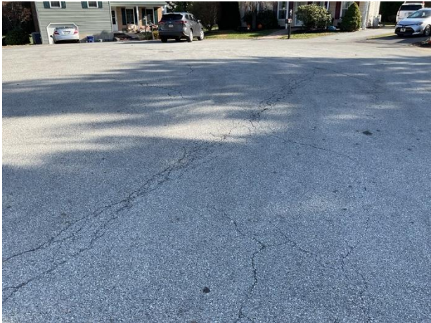
Pavement cracks on Essex Court
