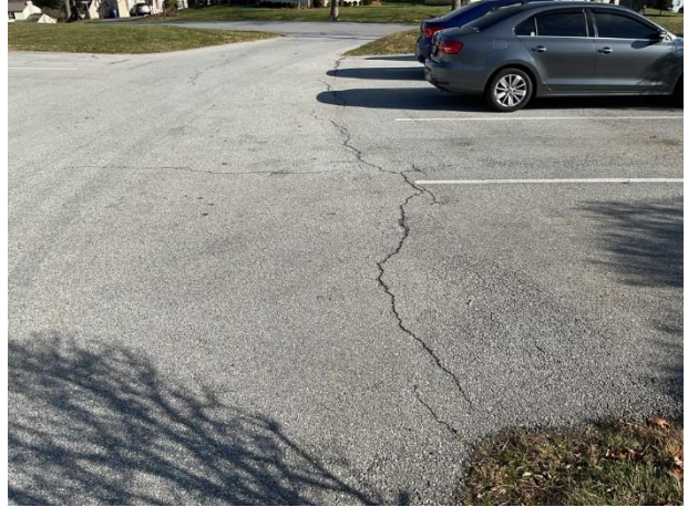
Longitudinal cracks on Hastings Court
