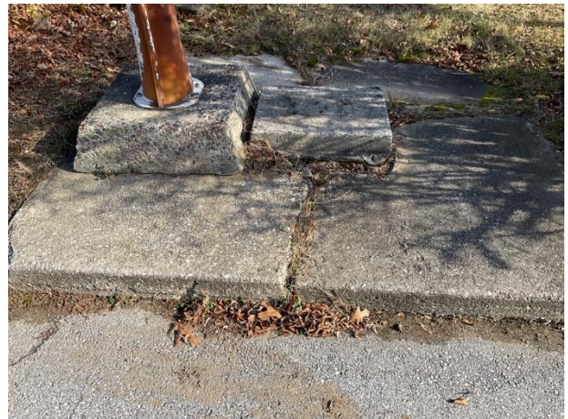
Cracks and deterioration
