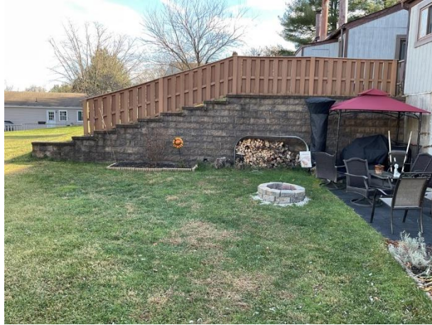
Masonry retaining wall
