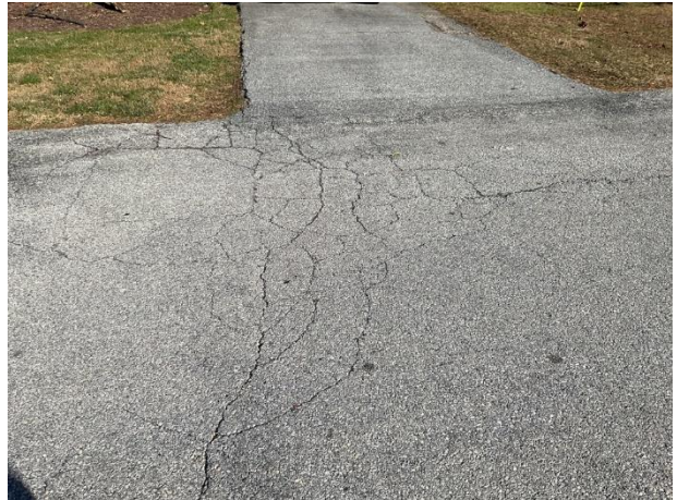
Alligator and edge cracks on Essex Court
