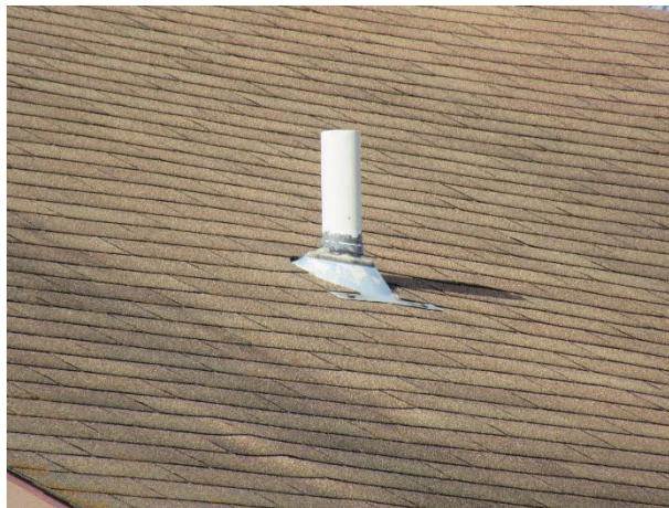
Waste pipe with metal boot
