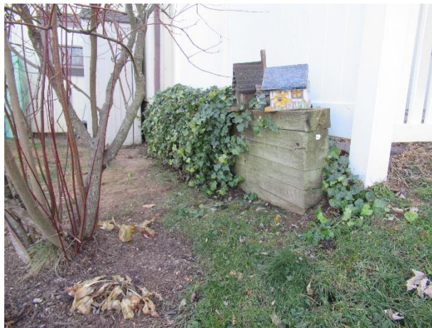
Timber retaining wall
