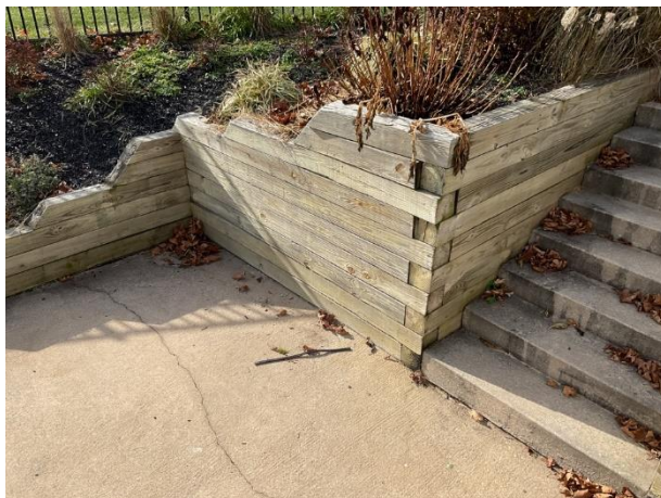
Timber retaining wall
