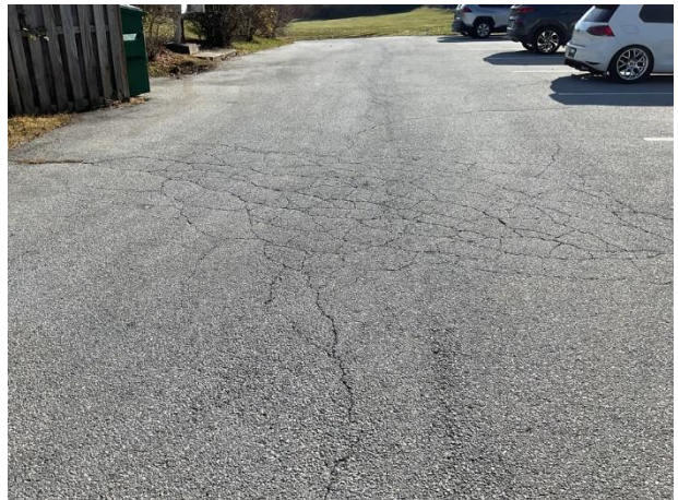
Alligator cracks on Hastings Court
