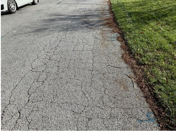
Pavement alligator cracks on Suffolk Court
