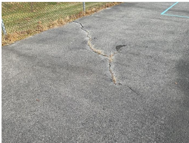
Surface cracks
