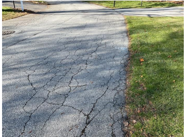
Alligator and edge cracks on Somerset Court
