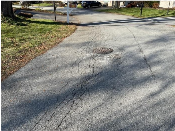
Alligator cracks on Somerset Court
