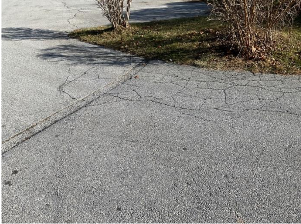
Pavement cracks on Hastings Court
