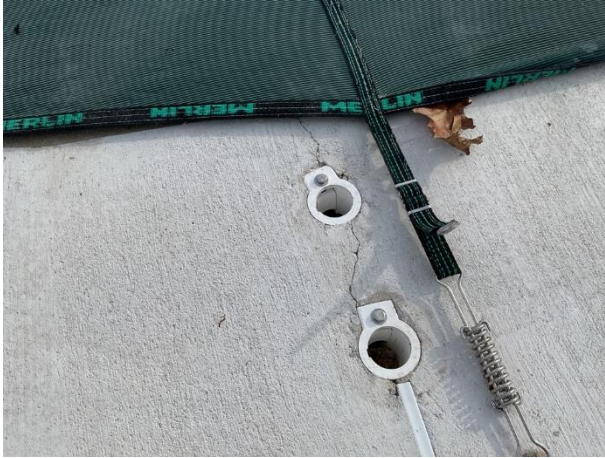
Concrete cracks
