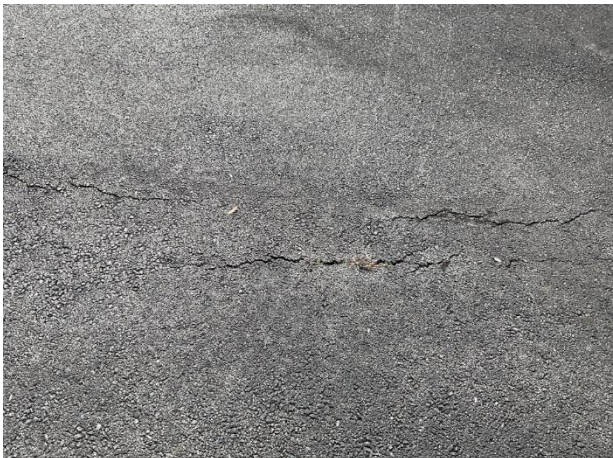
Surface cracks
